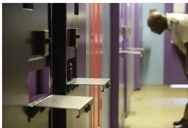
Left: Inside Ebongweni Supermaximum Prison. The door is solid steel with a shoebox-size slot through which food gets passed. (Image: Timeslive)
